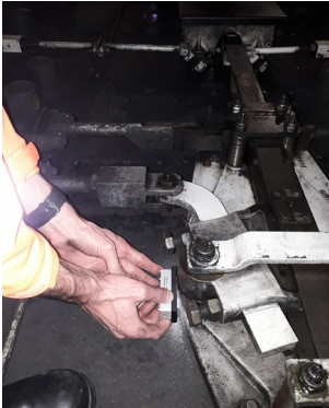
Mounting an enDAQ sensor track-side to monitor track vibration
